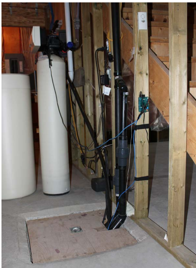
Figure 4. Finished Pit View
